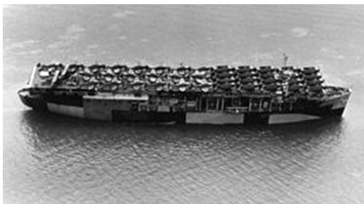
USS Long Island an Escort Carrier built in 77 days. It was made by converting a merchant ship to escort carrier. This is a feat only the Americans could do.
